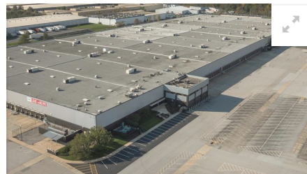
The former Giant warehouse at 7600 Assateague Drive in Jessup sold for more than $44 million.
